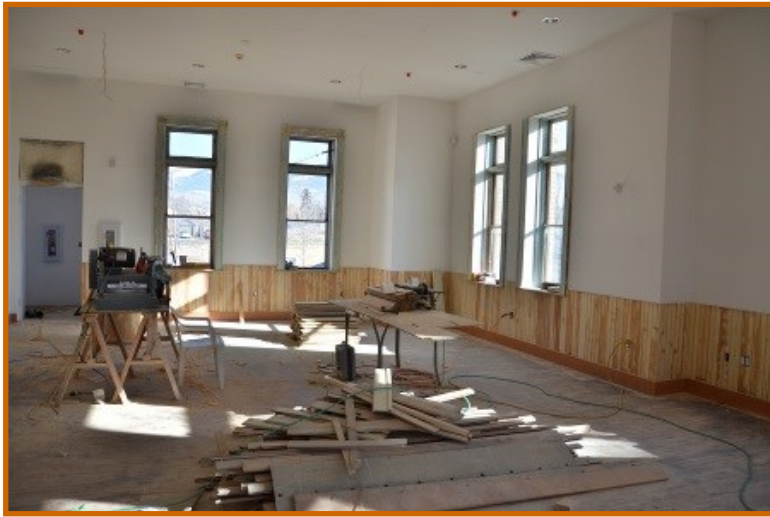
Main Floor—South East Room
