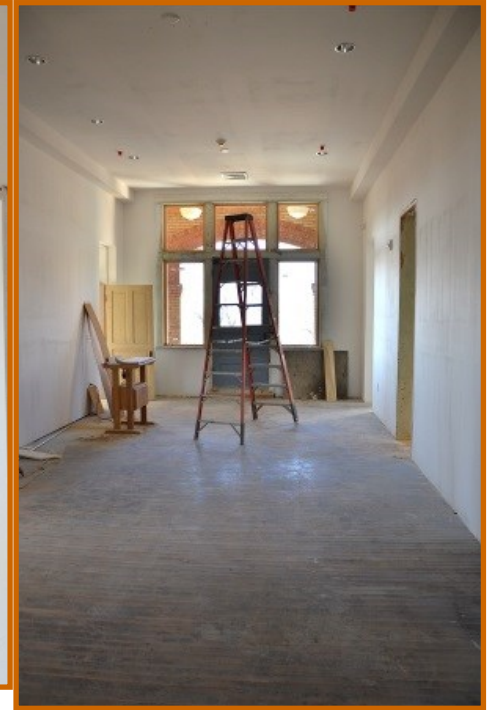
Second Floor Hall Looking West
