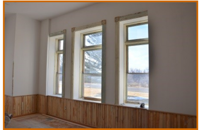
DUP Room—South West
